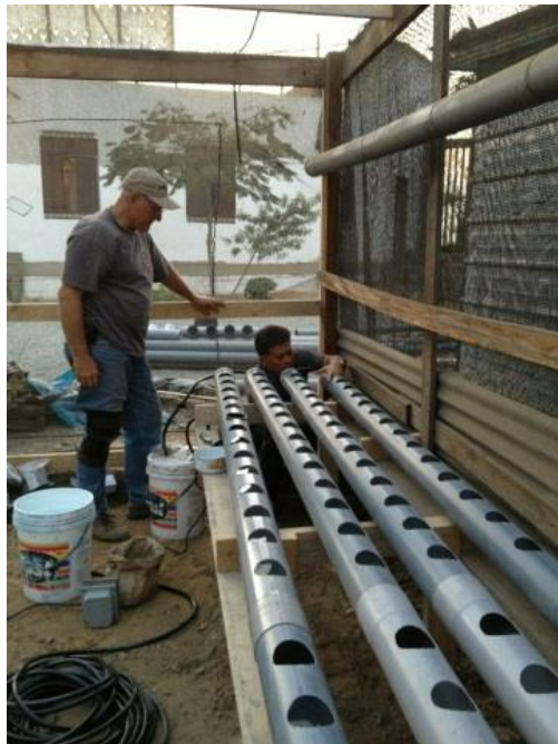
Figure 5. Water Pumps. Setting up the water pumps and filtration system. Used by permission of Zac and Mikaela Camp.
