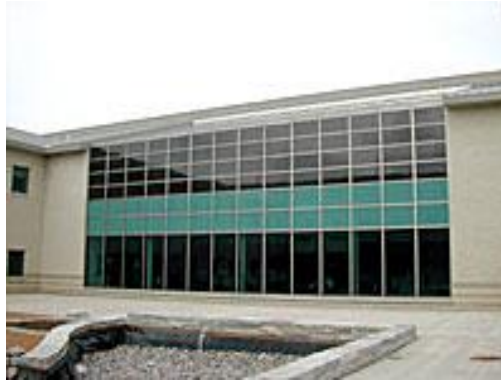
Figure 5: The finished photovoltaic wall at Mary Ann Cofrin Hall ( http://www.buildingsolar.com/visionglass.jpg ).
